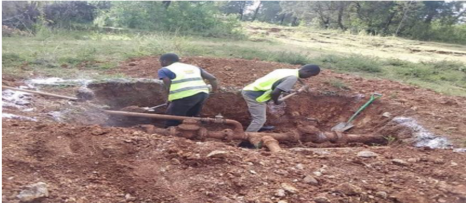
Exposing of existing water mains for rehabilitation.
